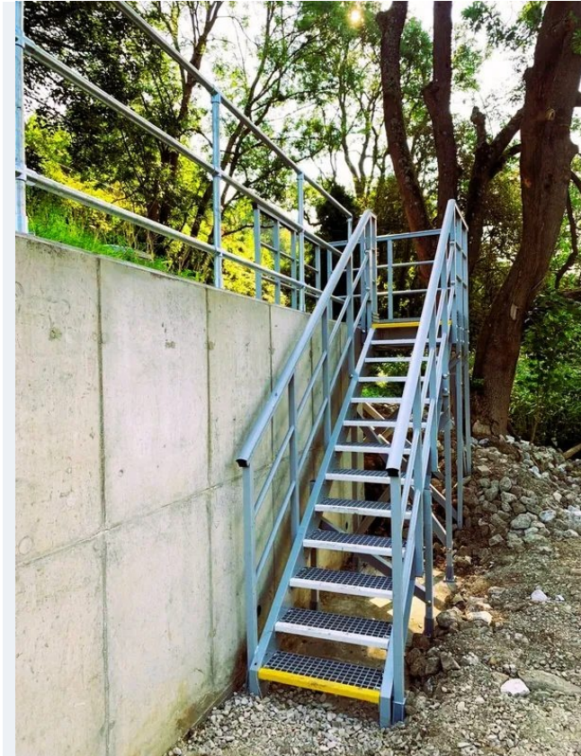
Modular GRP access steps installed beside the Hague Bar retaining wall.
