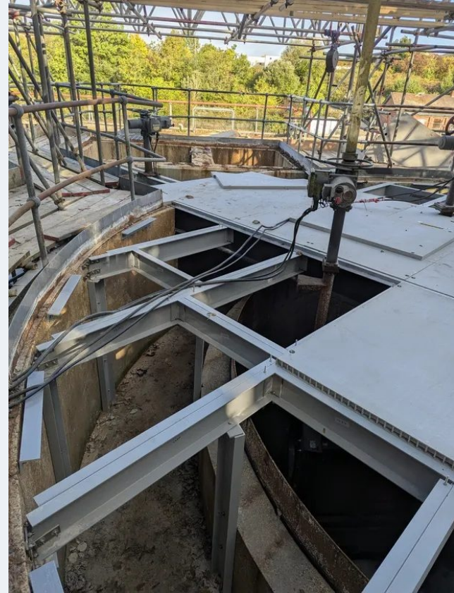
GRP support framework and chamber interface during the Southend works.
